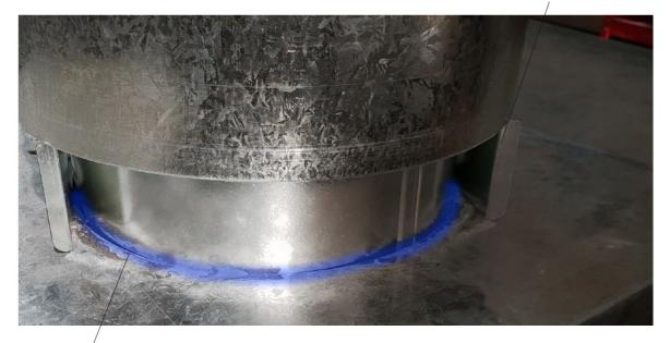
Use heat resistant sealant to seal 8" flue pipe to casing
