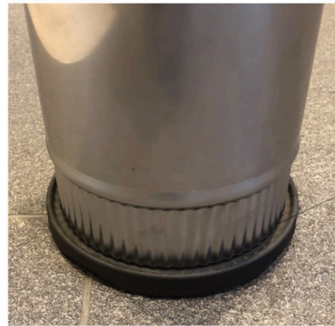
Flue seated correctly.
