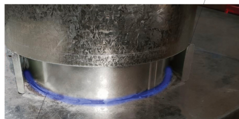
Second step in bracket stands off 10" flue pipe
